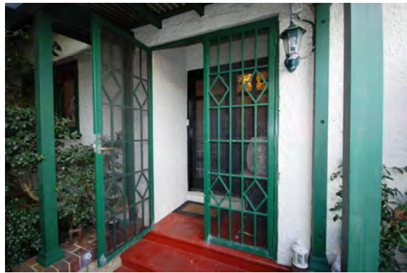
Figure 24: Entry recessed porch with security doors. The front doors to the house are behind. The timber pergola is a later addition but may be based on original details.
