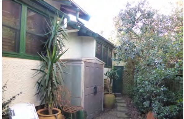
Figure 20: View of the rear of east elevation showing extended rear rooms with former garage in background.
