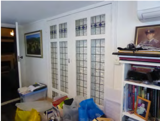
Figure 31: Timber double doors with leaded lights leading from the main bedroom into the front verandah, now the study.
