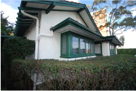
Figure 19: Detail of front bay window with leaded lights, boarded soffits, and exposed rafters.
