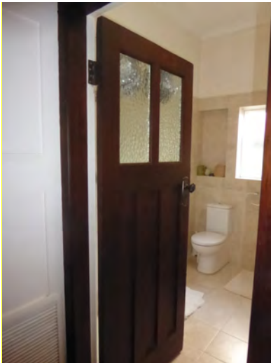
Figure 33: Original bathroom door obscure glazing to top panels.
