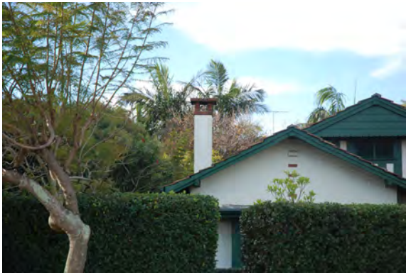
Figure 27: Detail of chimney and front gables.
