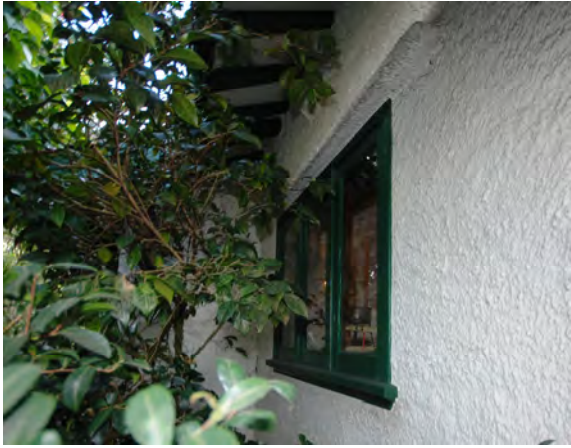
Figure 25: Typical timber casement window with roughcast hood above.
