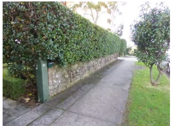
Figure 39: Original stone boundary wall along street frontage.
