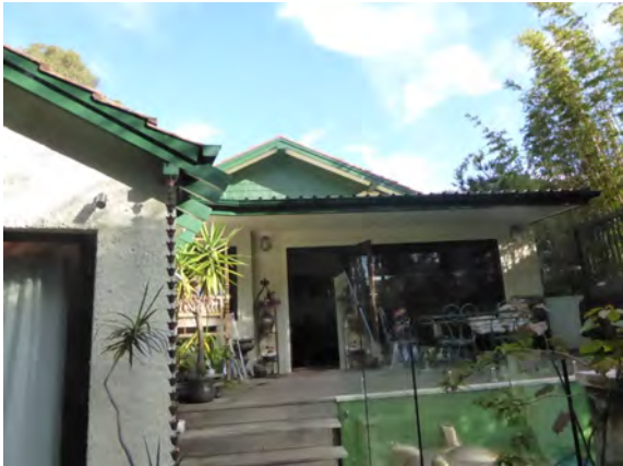
Figure 21: View of later addition Family room and deck, with former garage in foreground.
