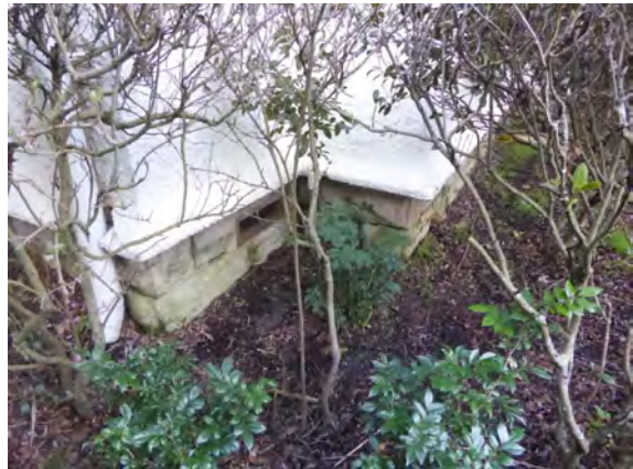
Figure 28: Detail of roughcast skirt over sandstone plinth at base of building.
