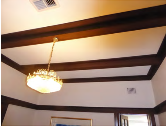
Figure 29: Timber ceiling battens and cornice in the Living Room
