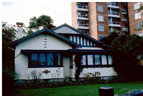
Figure 14: c.1991 photograph of No. 24 Cranbrook Avenue, Cremorne. Source: Australian Heritage Places Inventory/Register of the National Estate, Place ID. 17316
