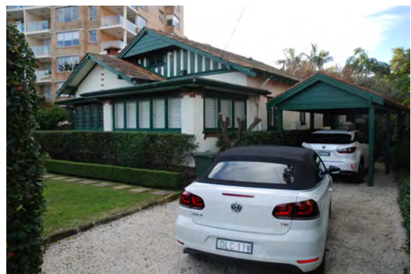
Figure 18: View of later addition carport on east elevation.
