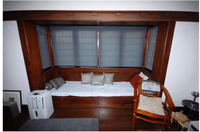
Figure 30: Timber joinery for the bay window in the Living room with plate rail above.
