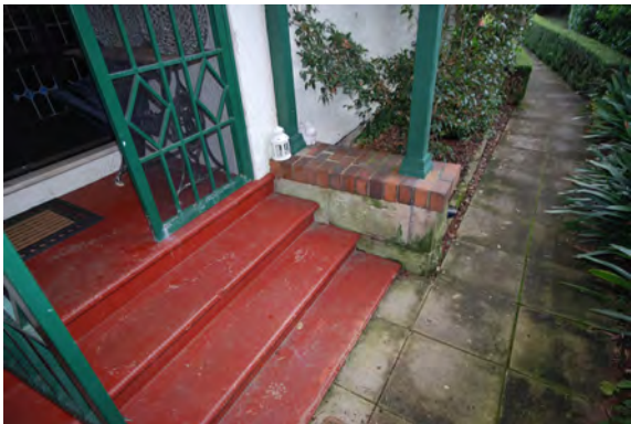
Figure 23: Front concrete steps with sandstone side walls with brick capping.
