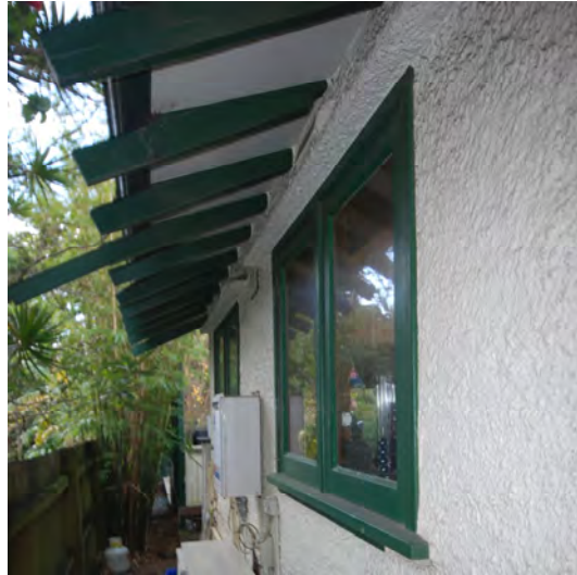
Figure 26: Typical timber casement window with exposed over-sailing rafters above.
