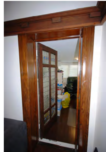
Figure 35: Door from Living room to front verandah with leaded lights.
