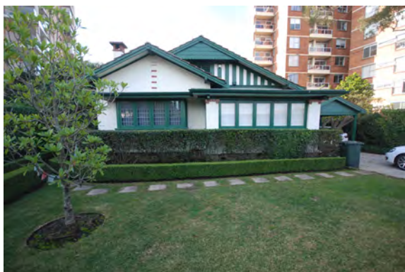
Figure 17: Front elevation of 24 Cranbrook Avenue with enclosed front verandah and double gables.
