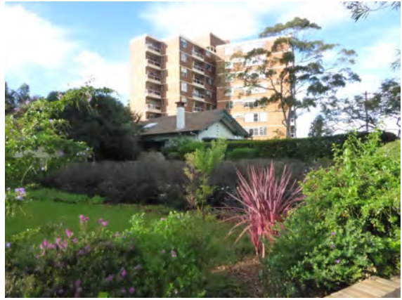
Figure 22: Roof of the house with front gable and chimney as seen from Cranbrook Avenue.
