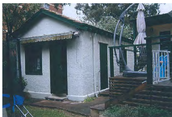
Figure 16: View of the rear and side elevations of the garage in 2010 prior to its conversion into a cabana in 2011. Source: North Sydney Council, DA473/10
